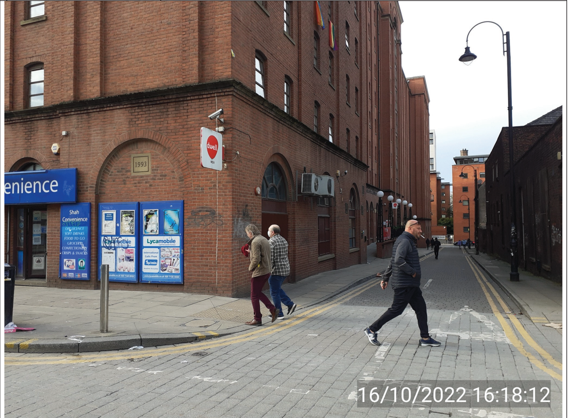
097705: Shah Convenience Store, Student Village, Lower Chatham Street, Manchester M1 5SS (Lower Chatham Street elevation)
